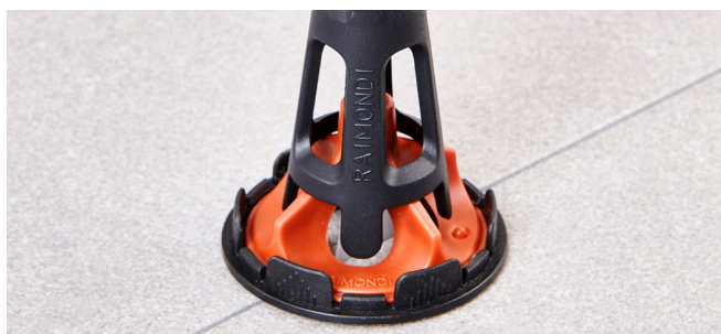
TWIST CAP ONTO CLIP
