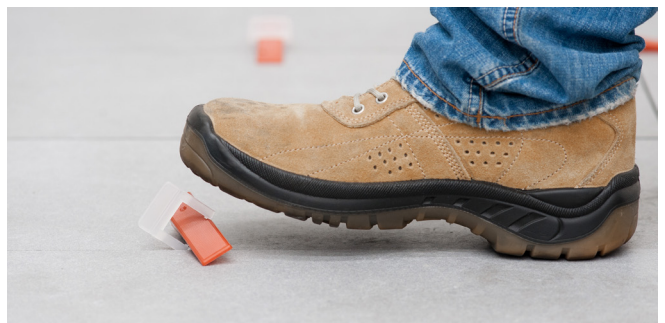
REMOVE CLIP AND WEDGE
