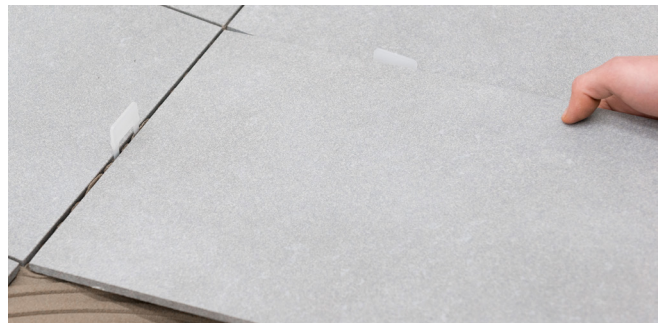
INSTALL & EMBED TILE
